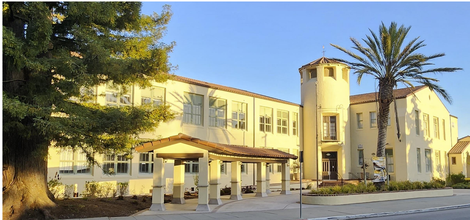
View from King Street: Windows coming this summer
